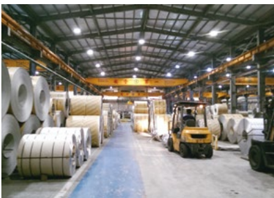
CAP1200 Access Point wireless deployed in the factory.
